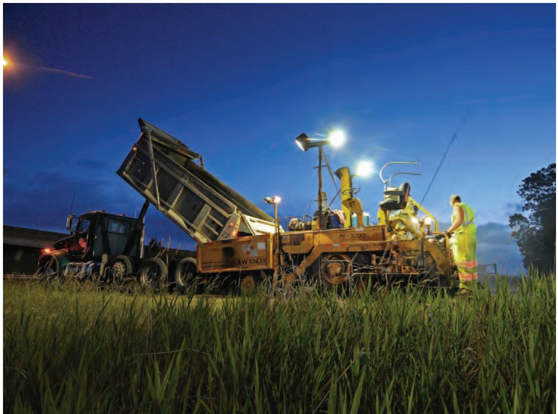
Photo by David Gonzalez, Minnesota Department of Transportation
