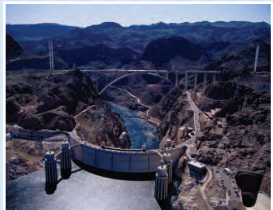
Photo courtesy of Federal Highway Administration
