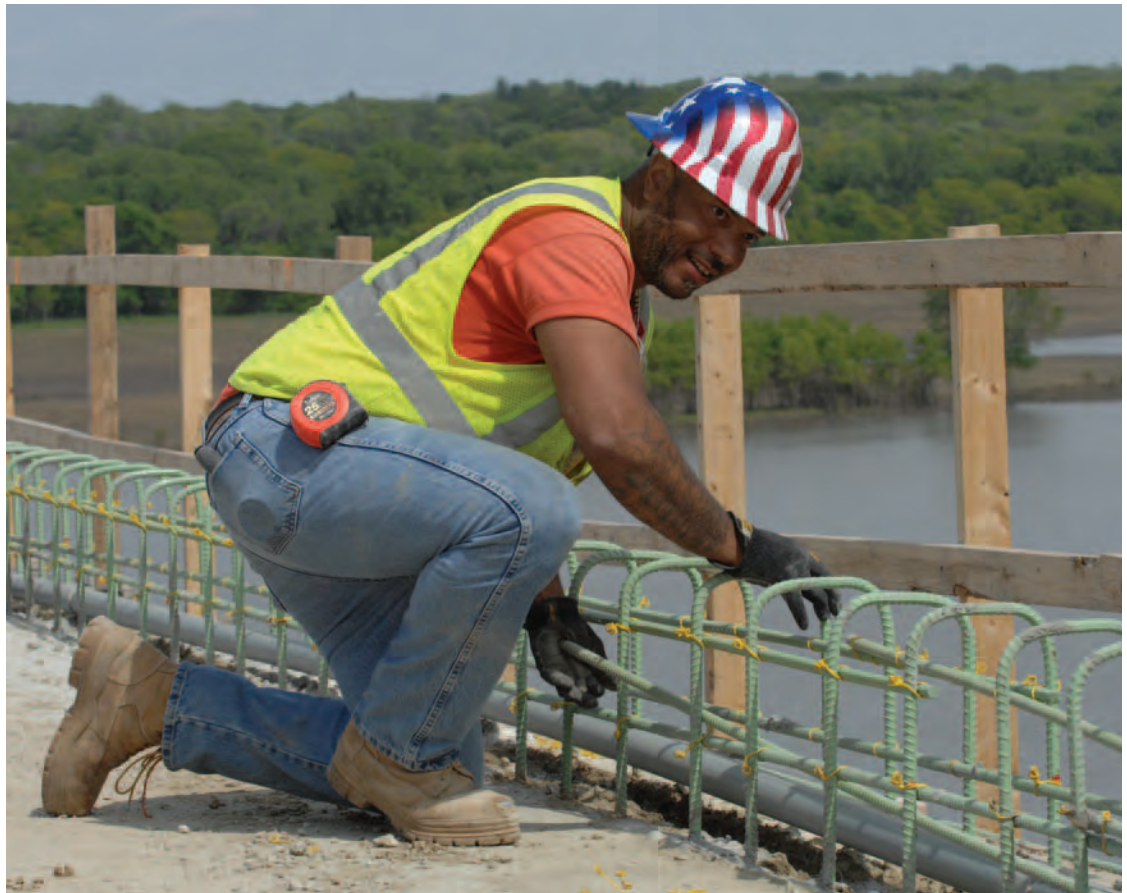
A construction worker installs reinforced steel on the Des Moines River bridge, connecting Boone and Madrid, IA.
