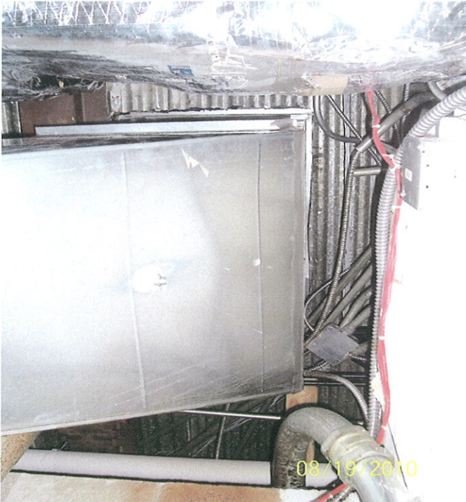
PICTURE #7-ROOF DECKING IN ELECTRICAL ROOM ON FIRST FLOOR-AREA HAS SUSTAINED SEVERAL WATER LEAKS
