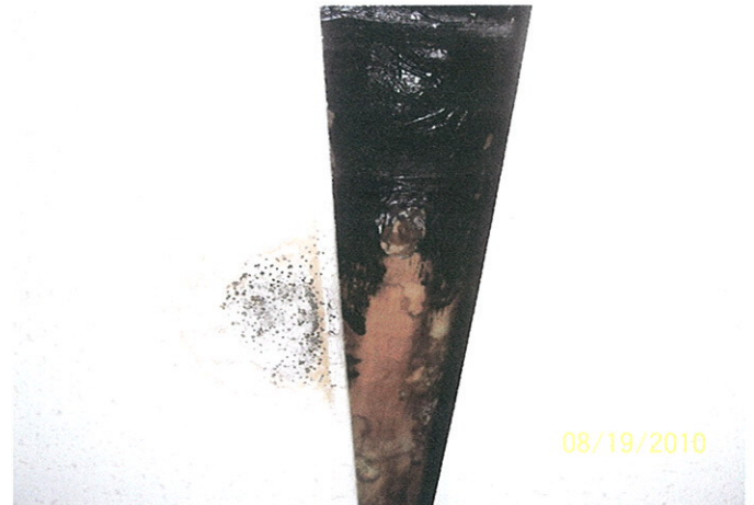
PICTURE #8-WATER DAMAGED CEILING TILE AND FUNGAL GROWTH IN BACK CORRIDOR OF FIRST FLOOR-WATER DAMAGE IS FROM PIPE CONDENSATION
