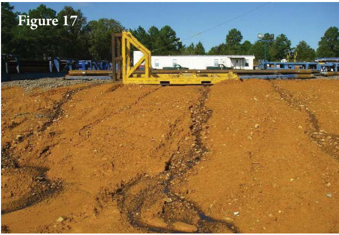
Drilling fluids leaking and running off of a well pad will end up in a nearby lake or stream.
