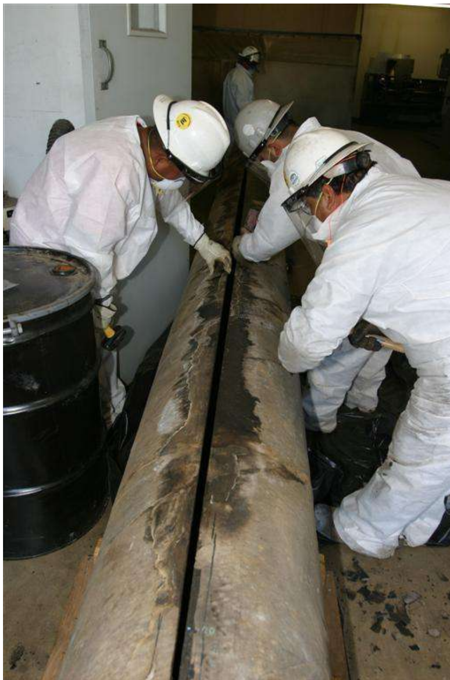
The photograph displays the careful hand removal process of the coating adjacent to the crack.
