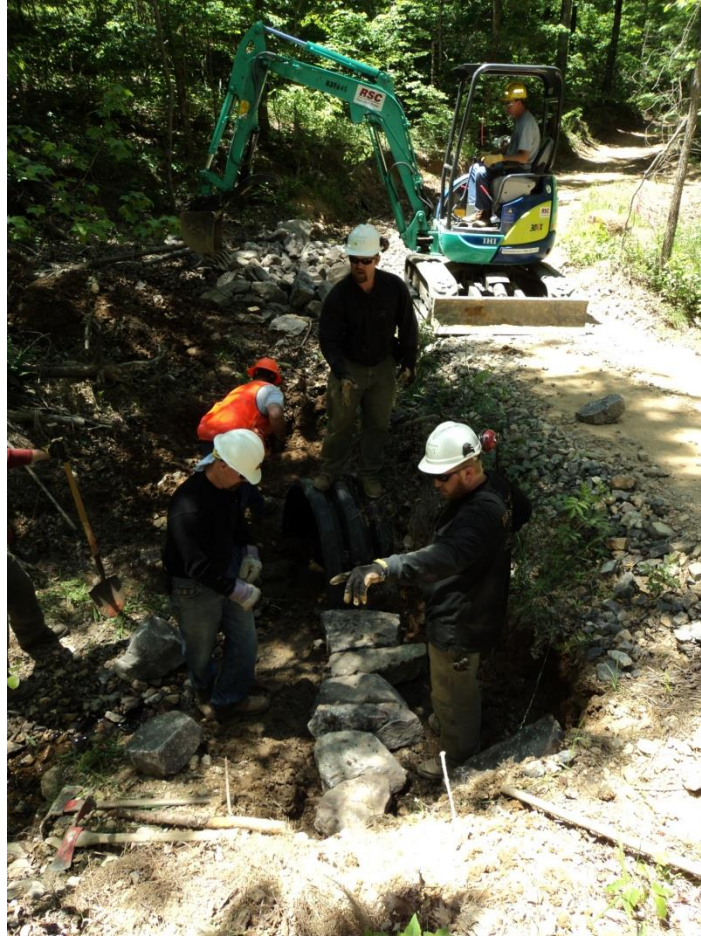
Figure 2. Ouachita ATV Club, Trails Unlimited, and Ouachita NF employees installing an arch culvert to reduce sedimentation (improve water quality).
