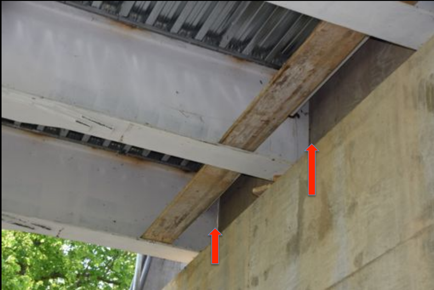
Beam resting on north abutment wall
