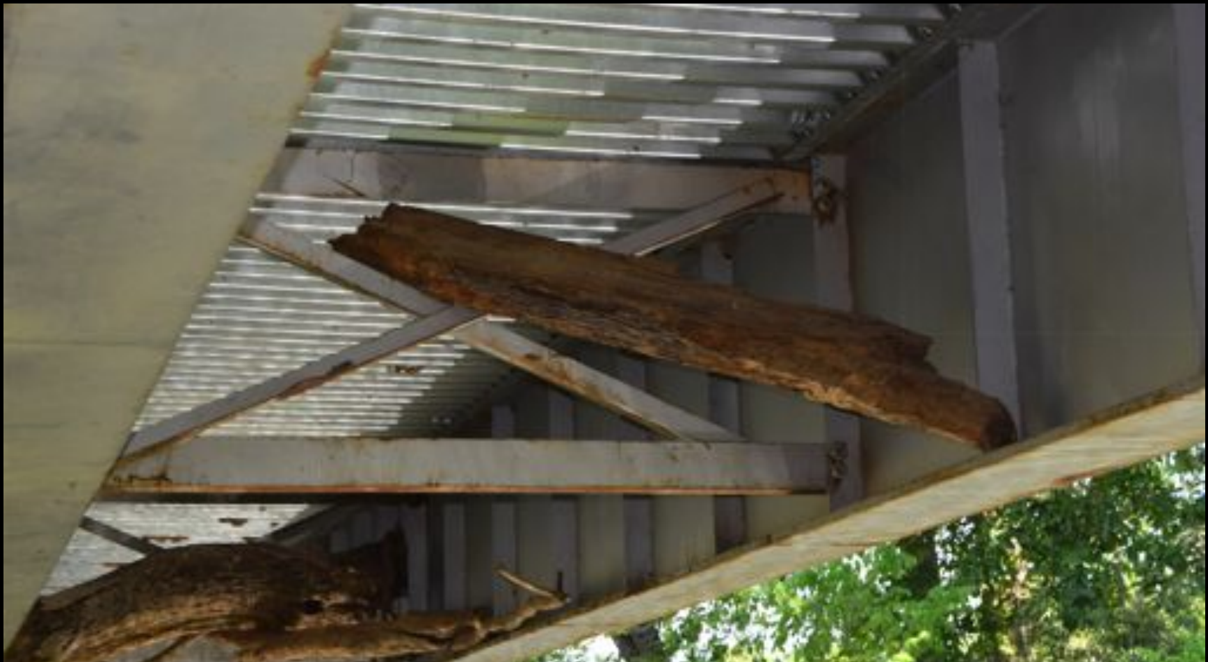
Logs in steel beams under 62 bridge
