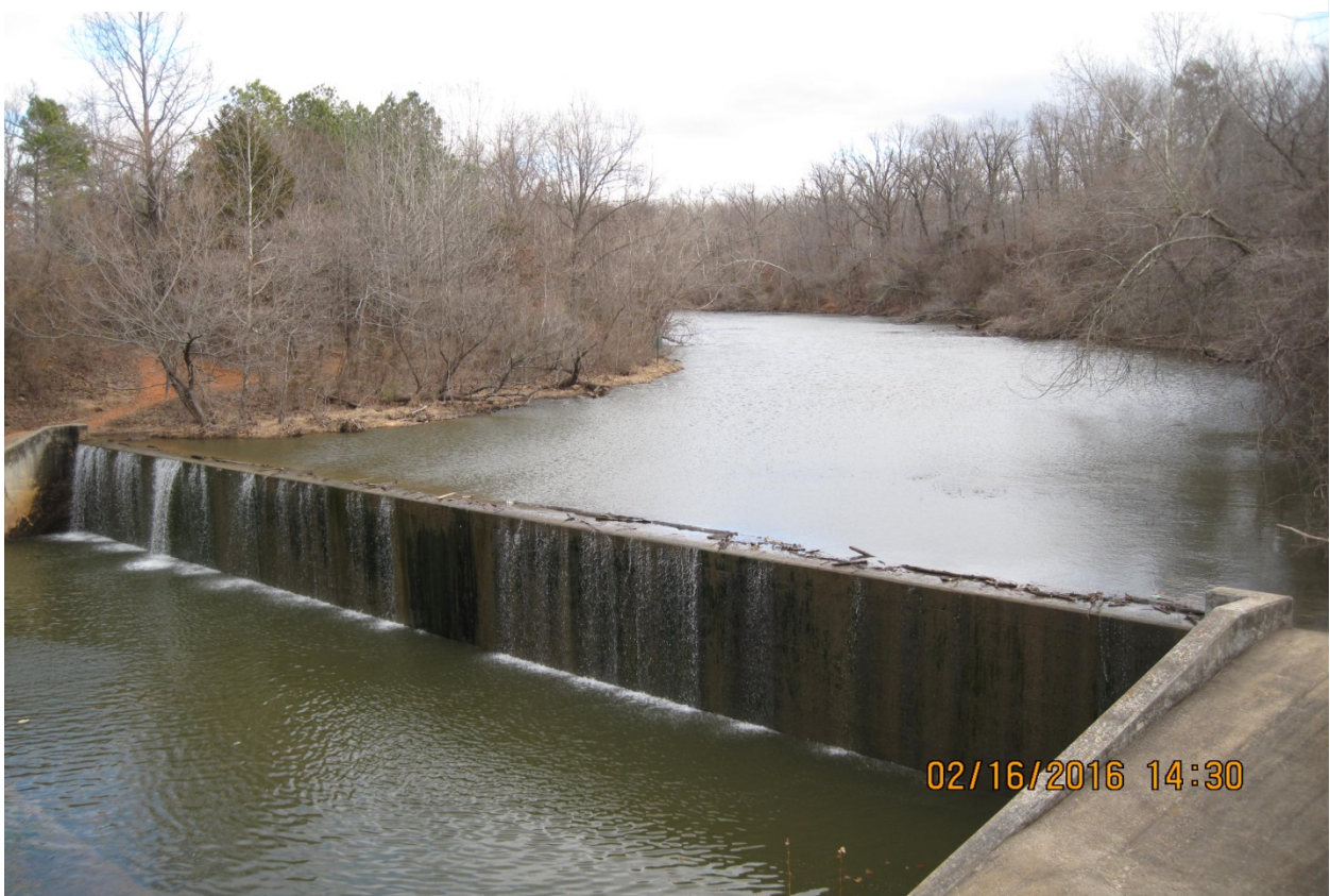
Figure 3 Spillway crest
