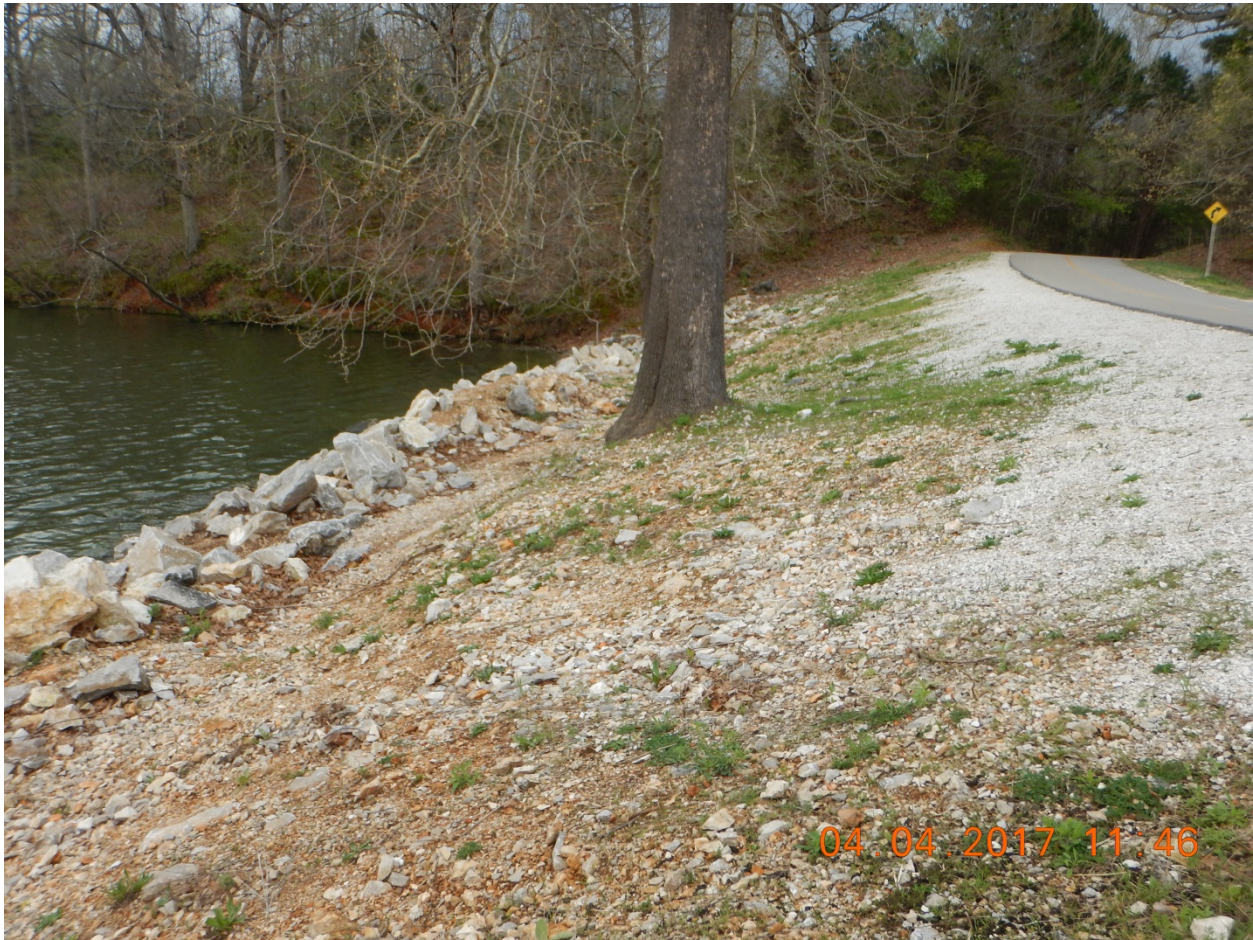
Figure 3. Signs of erosion on the lower portion of the upstream slope above the rip-rap line.
