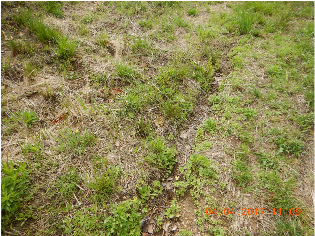
Figure 5. Ruts on downstream slope of dam.
