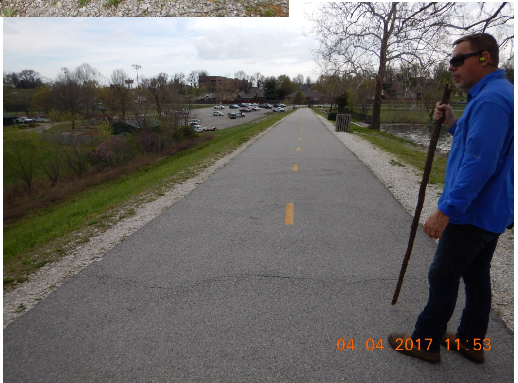
Figures 1 & 2. Large trees growing on upstream slope. Cracks forming on crest of dam caused by root systems of large trees.
