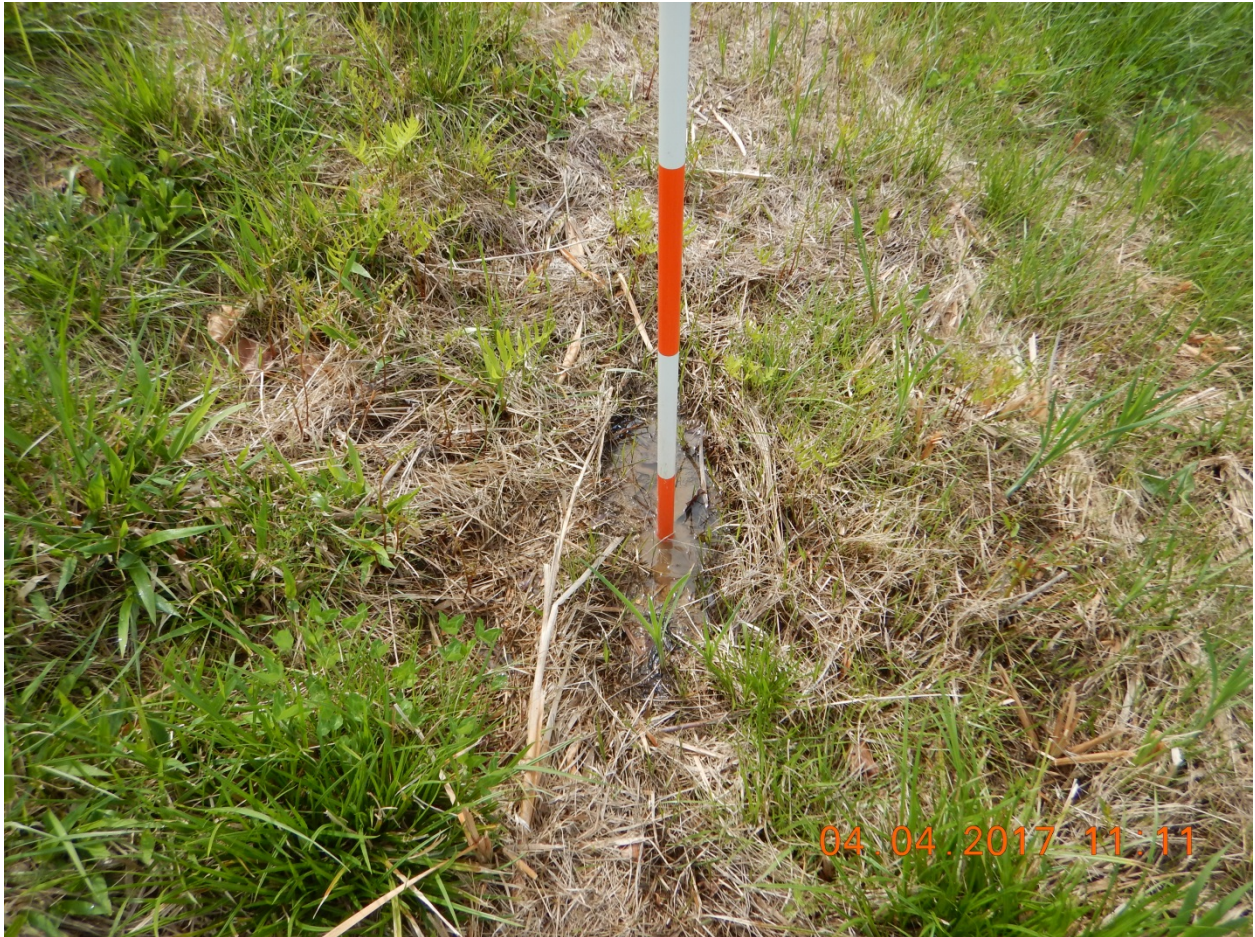
Figure 4. Seepage on downstream slope of dam.
