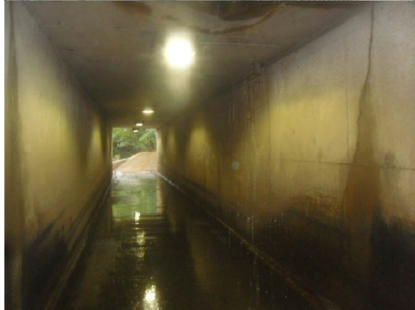
EXISTING TRAIL CONDITIONS - WET ALL OF THE TIME
