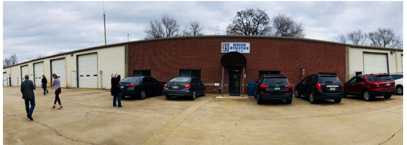
Former City of Bentonville utility building
