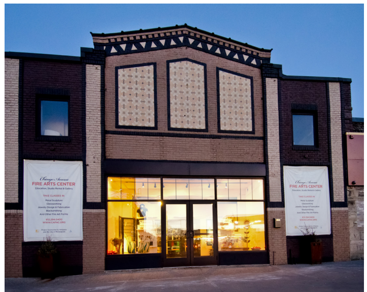
Chicago Avenue Fire Arts Center (CAFAC), Minneapolis, MN
