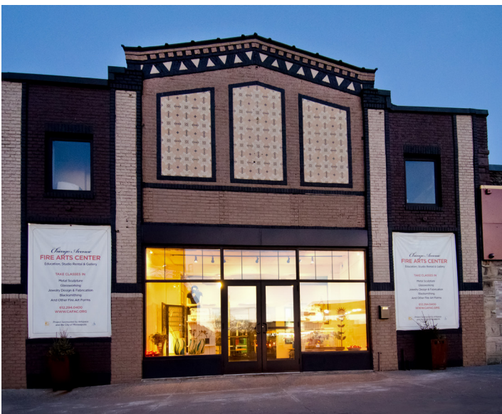
Chicago Avenue Fire Arts Center (CAFAC), Minneapolis, MN
