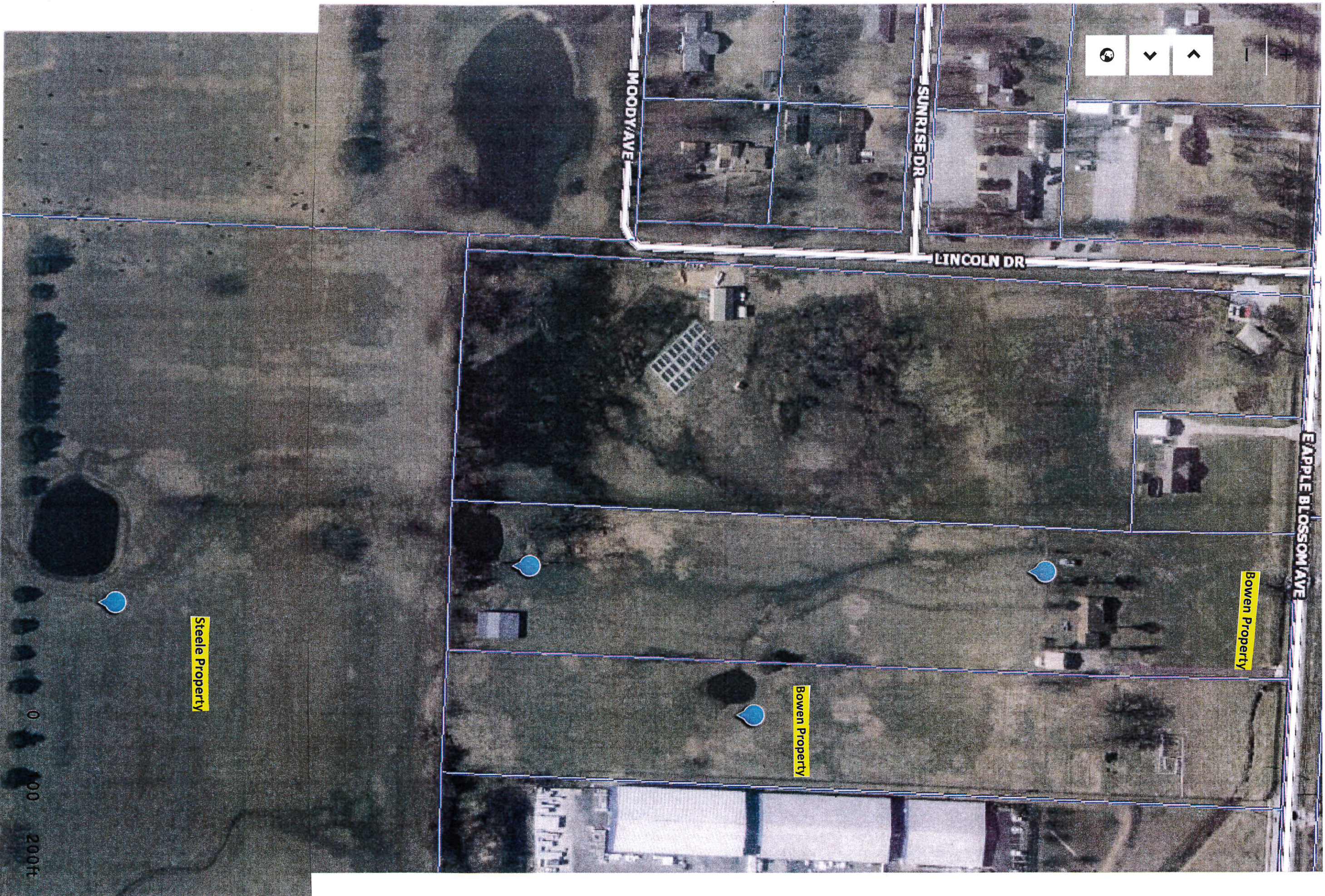
The aerial image above shows the ponds located on each neighbor's property. The blue balloons mark each pond. During rain events runoff from these three ponds converge together in the Bowens hay field and side yard swale that form a pathway into the drainage ditch on Apple Blossom Street. The dark green path shows the trail from each pond to the West side yard of Bowen property.
