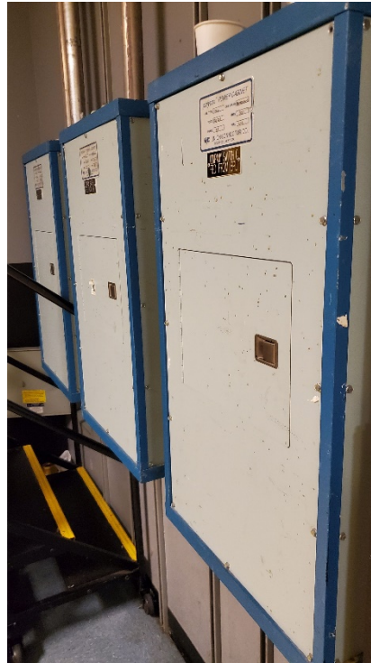
Figure 5: Panels at Ballroom
