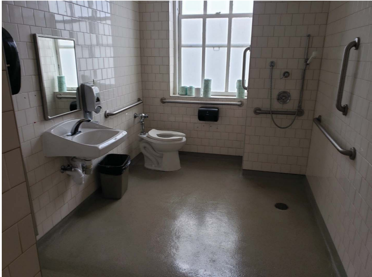
RENOVATED RESTROOM ON 2 ND FLOOR
