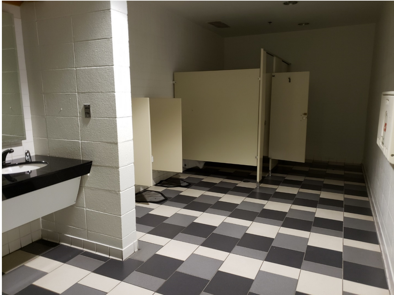
TYPICAL RESTROOM OFF GOVERNOR'S HALL
