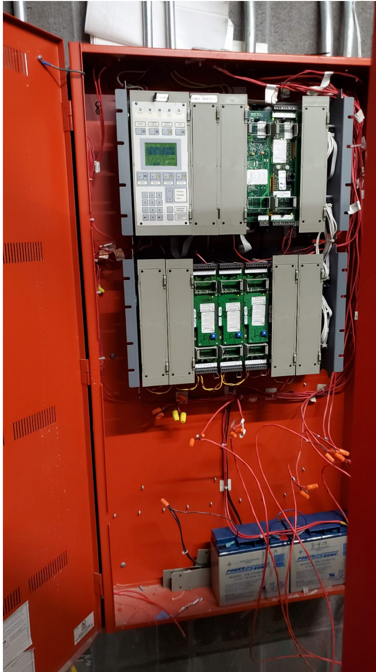
TYPICAL FIRE ALARM PANEL
