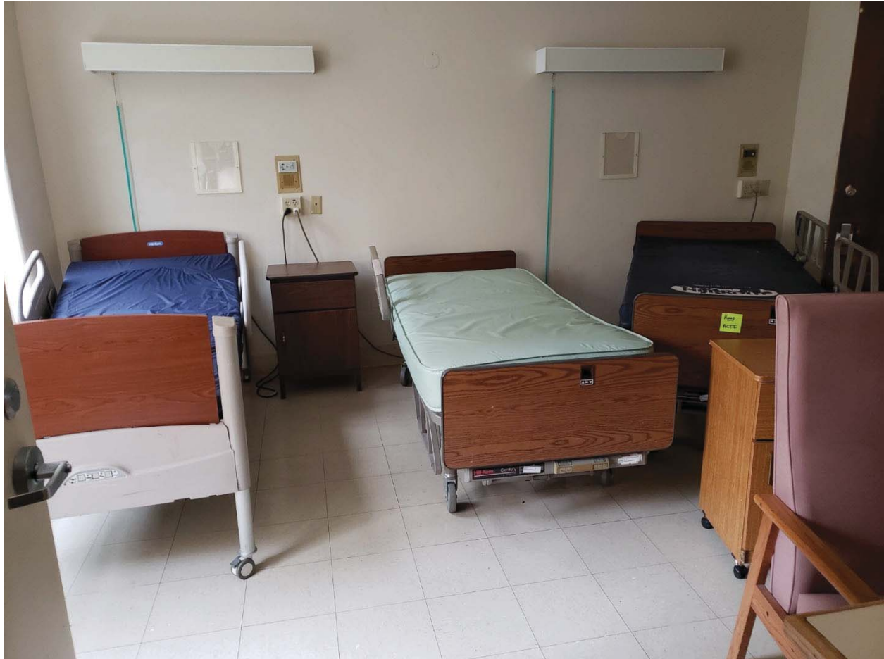
PATIENT ROOM WITH ELECTRICAL OUTLETS ON WALL
