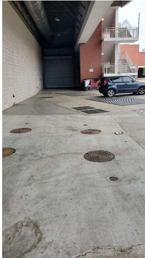
Figure 2: Temp Gen Location at Apron
