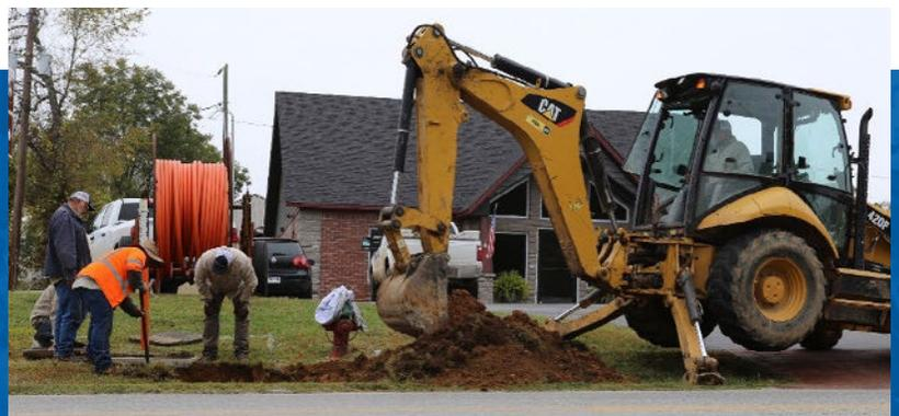
Running underground conduit for fiber infrastructure (Photo courtesy of Yelcot)
