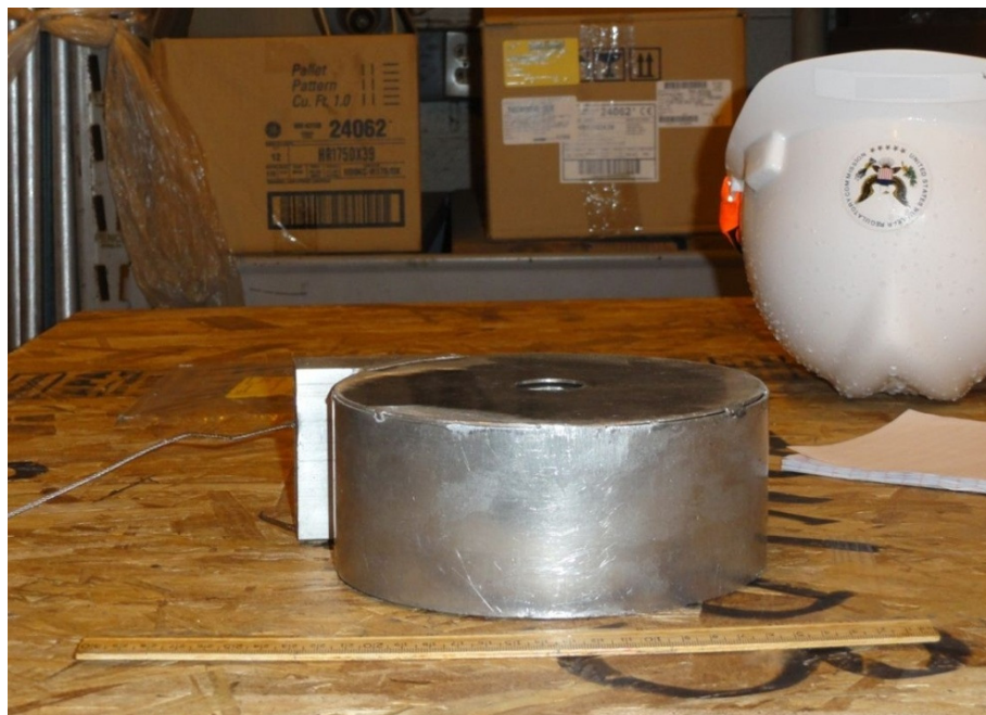
The SRM cable take-up cartridge at the Perry plant.
