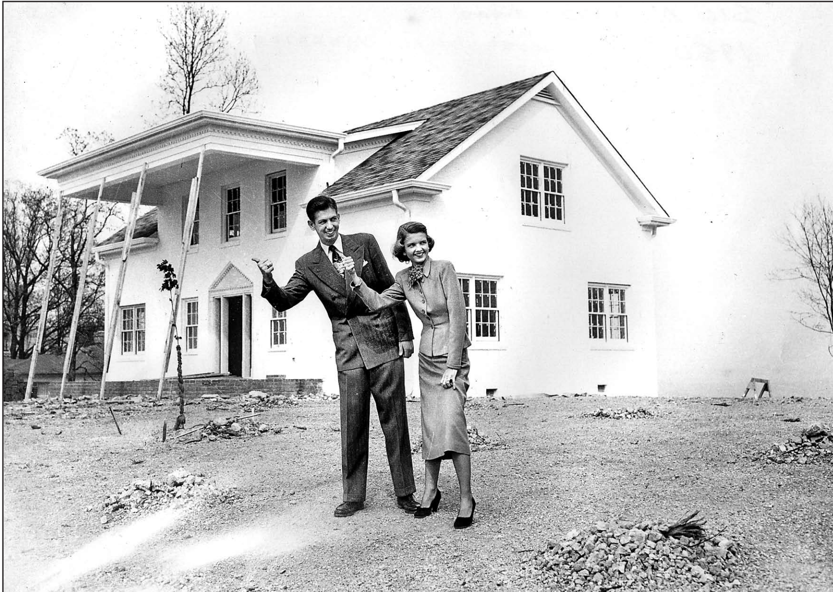
Lee Anderson and his wife, Betsy, stand outside their house while it is still under construction in 1950.
