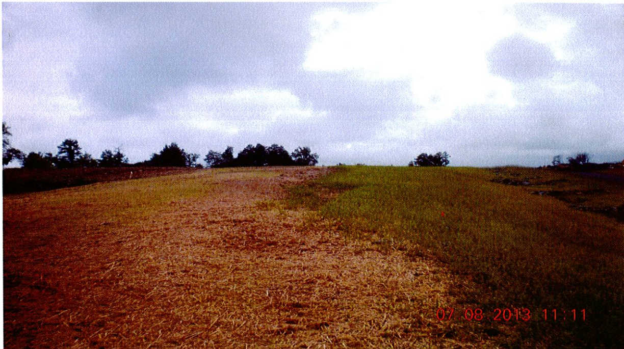
Photograph 2: Photo of the same private inholding showing the flat area above the steep slope in the above picture. Although seed and straw has been utilized, this area and any others with recent stabilization attempts must be monitored to ensure proper vegetative growth is established. Any changes in the grades of this area should be reflected in your amended SWPPP.
