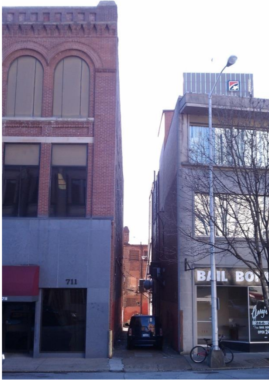
Alley from Cherry to Site (looking west)
