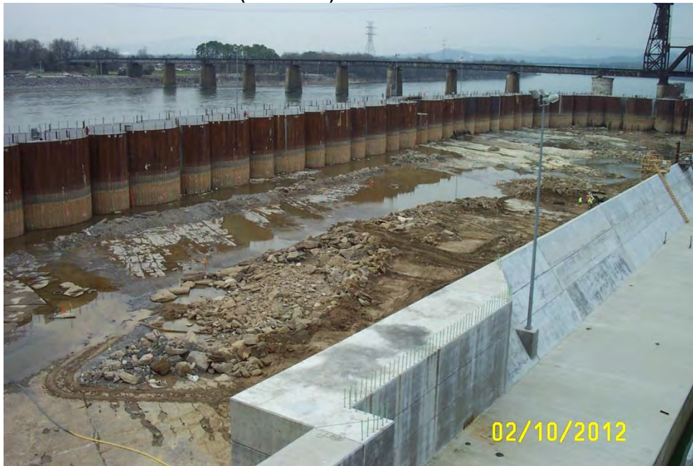
Overview of cofferdam (dewatered)
