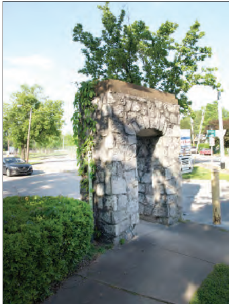
A. Original Entrance Pillar at Corner of Blackford and Central.
