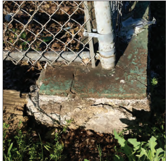
D. Detail of Southwest Corner of Tennis Court.
