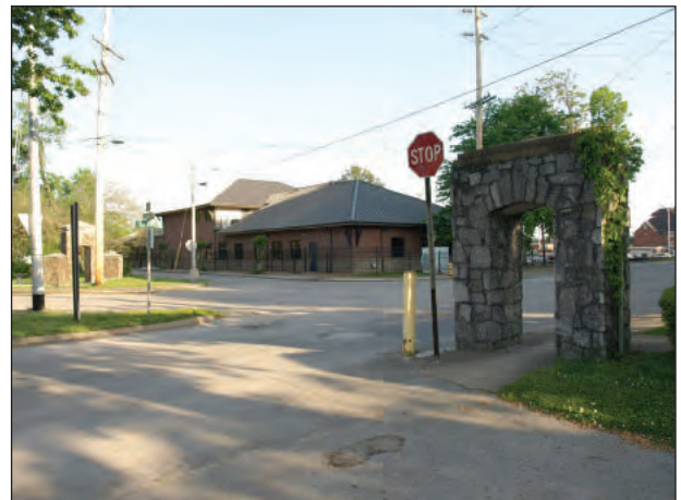
D. View of Current Entrance to Former Park Road Showing Existing Road Width Near Pillar.
