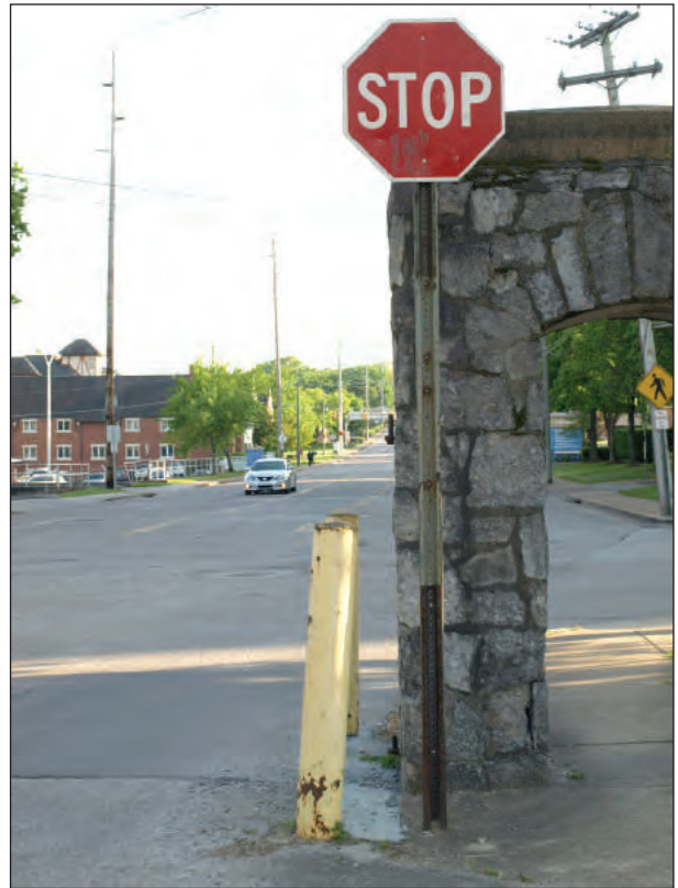
B. View South Showing Close Proximity to Existing Road.
