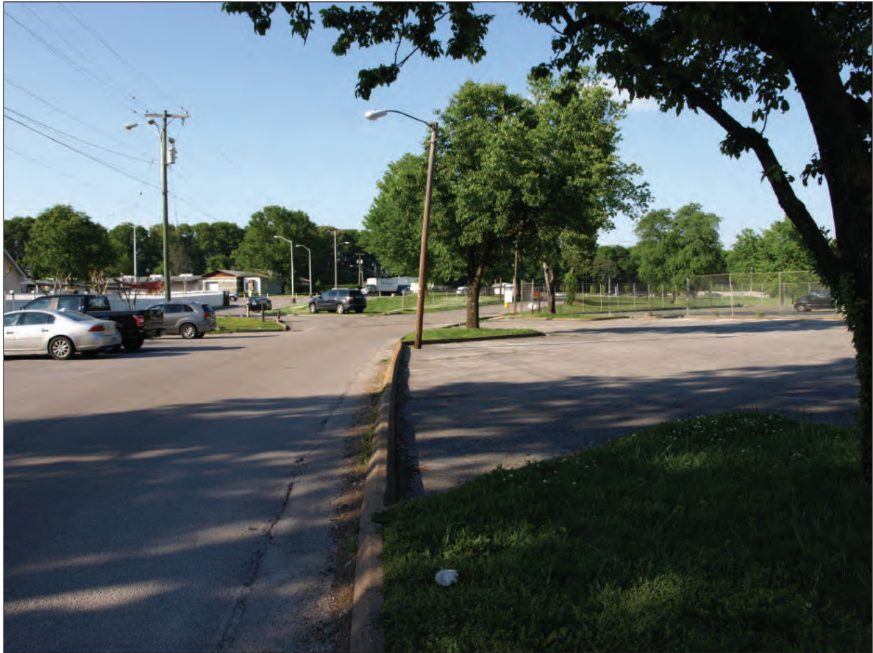
Figure 20. Visual Changes Resulting from Installation of Parallel Parking
