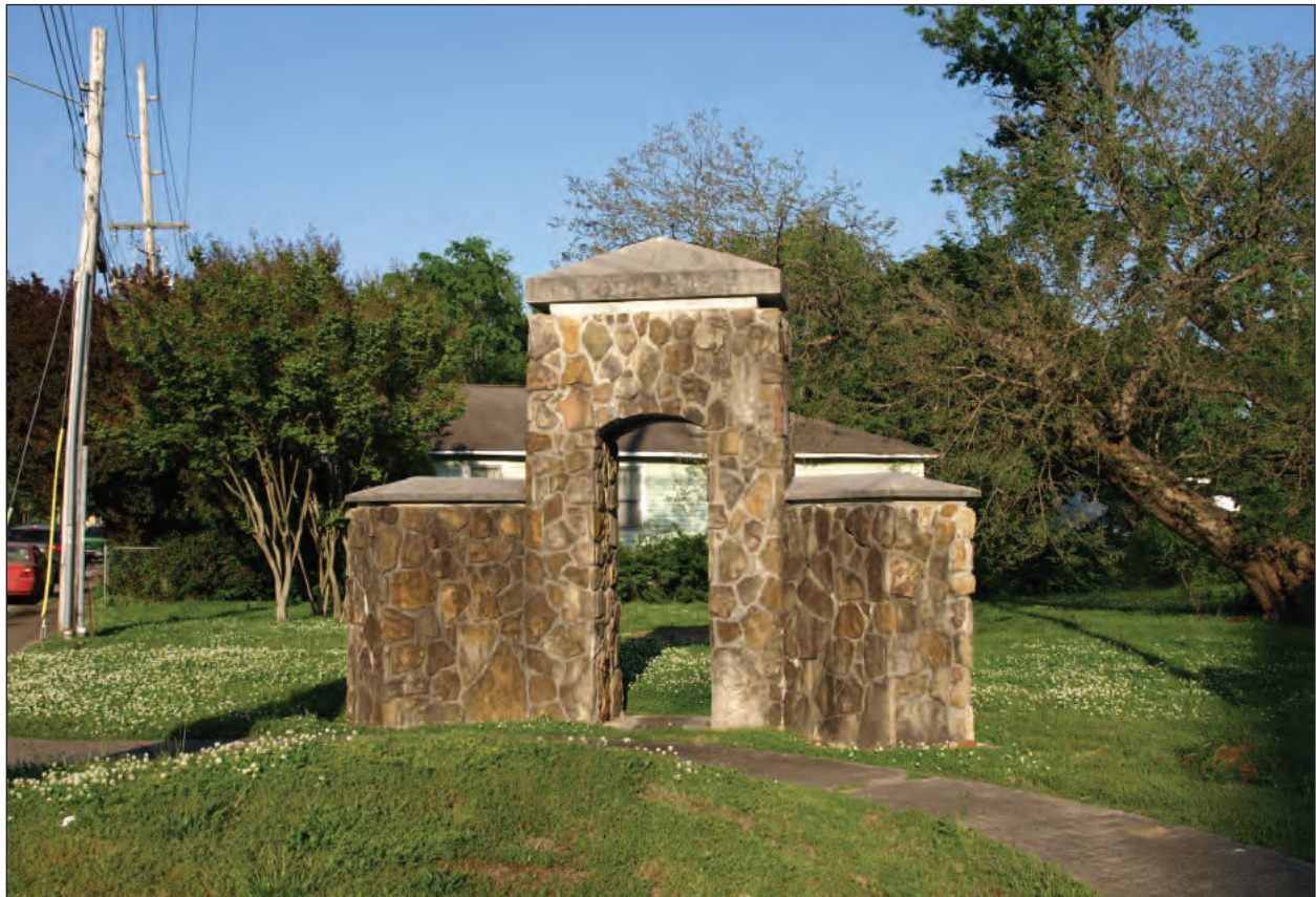
C. Commemorative Pillar on Blackford Street and Cleveland Avenue.
