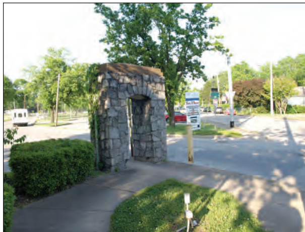
C. Grass Area and Pillar inside the NRHP Boundary and Pillar that would be Affected in Alternative K3.
