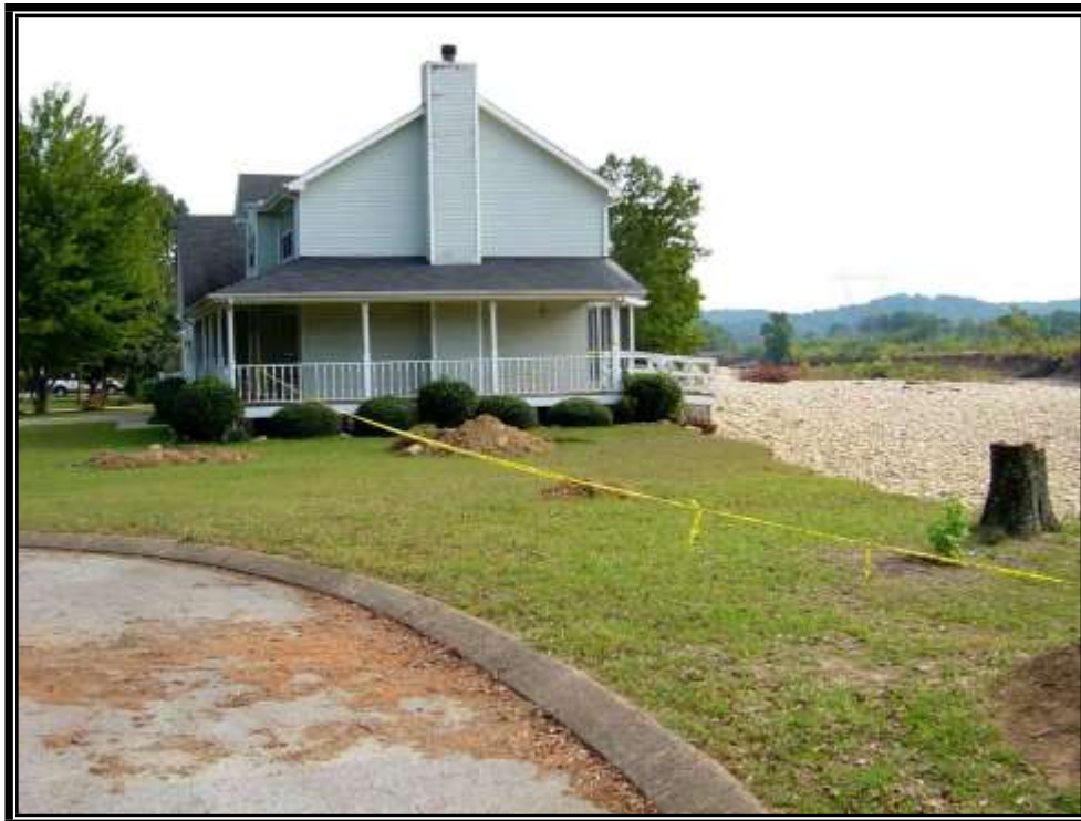
Streambank erosion in Willow Creek Subdivision on North Chickamauga Creek
