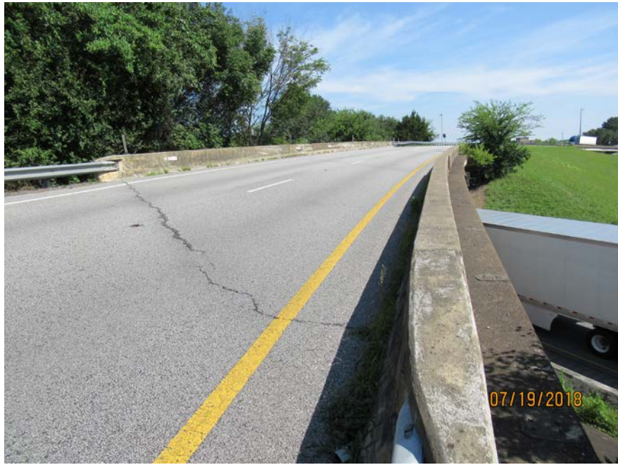
TOP OF DECK - AHEAD - SOUTHBOUND
