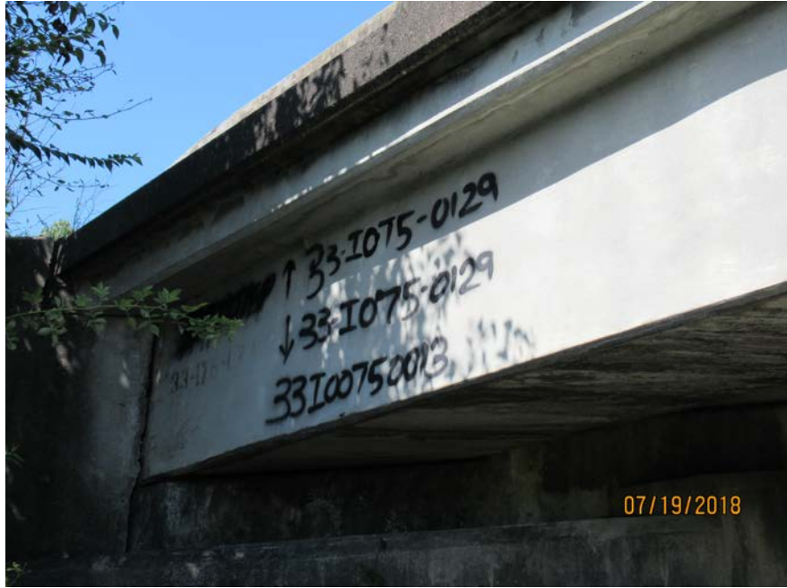
BRIDGE NUMBER - SPAN 1 - BEAM K
