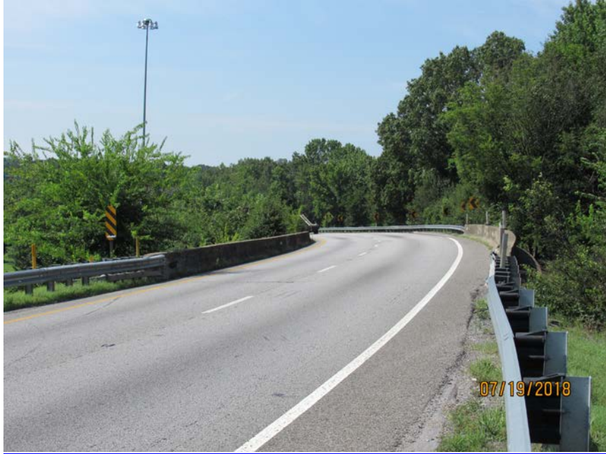
TOP OF DECK - BACK - SOUTHBOUND
