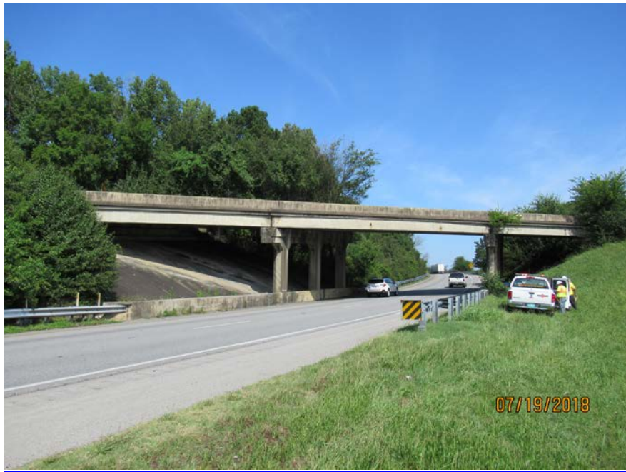
SIDEVIEW - RIGHT - AHEAD ON I-75 - NORTH
